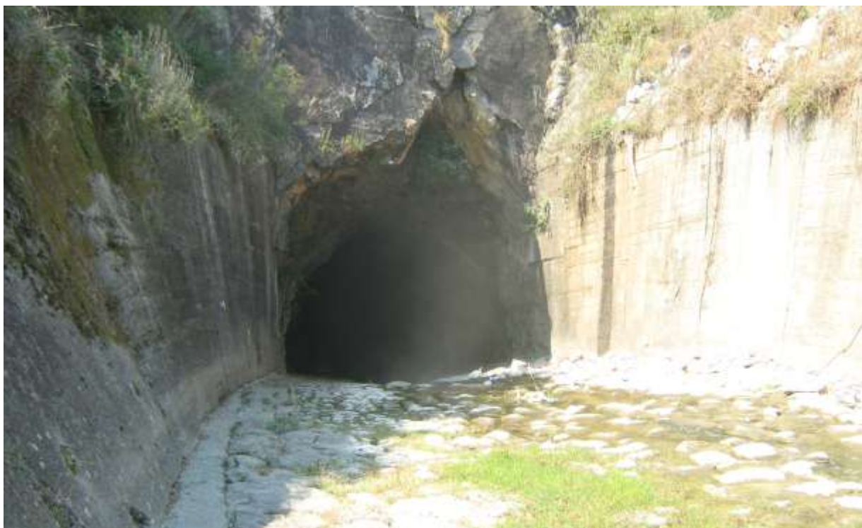
Prilog br. 27: Ulaz Rikavca u tunel
